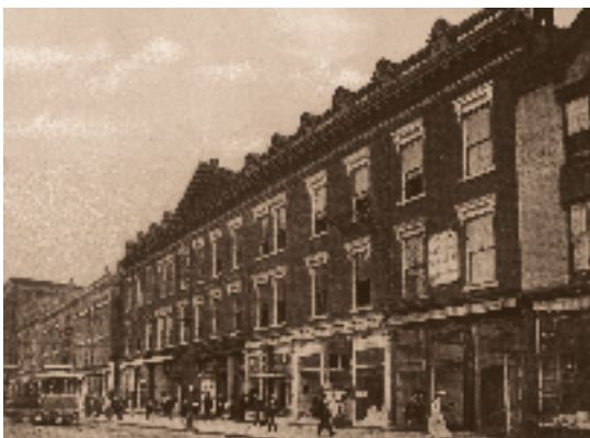
Academy of Music Building on Main Street. Burnt down in April 1930 and the Selden Arcade was built on the same site the next year.
